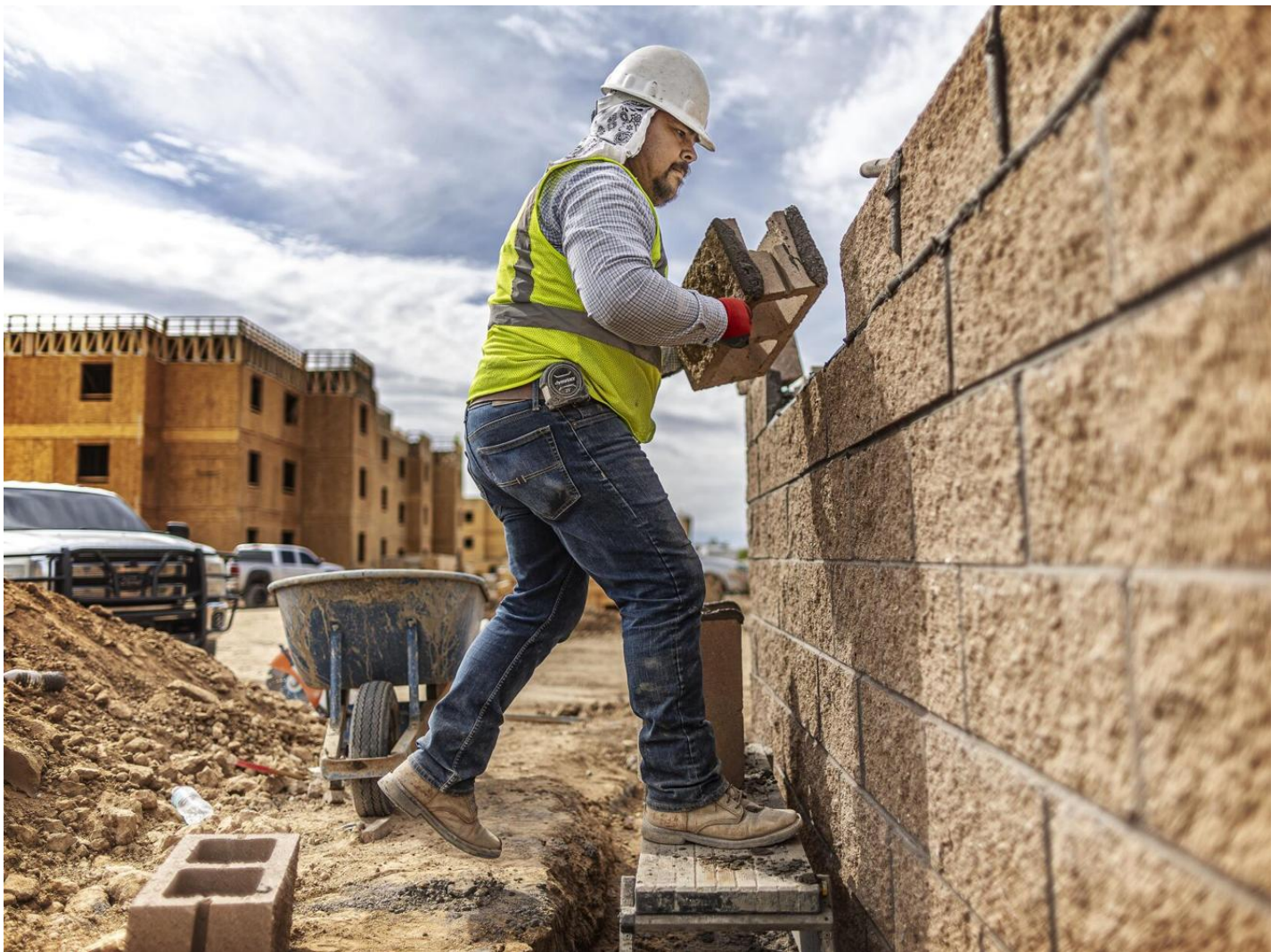
Pablo Ramirez lays block for a dumpster enclosure as construction continues Wednesday at the Cresta Ranch Apartments on Cerrillos Road near Interstate 25. The complex will be income-restricted, adding to the city's affordable housing supply.
